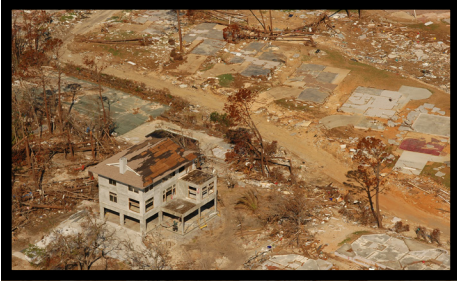
ICF home left standing and surrounded by rubble in the aftermath of Hurricane Katrina. Source: Insulating Concrete Forms Association, "ICFs Stand Up to Storms"
