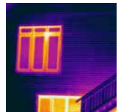
Thermal image of a home built with ICFs.
